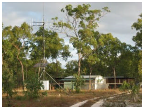
Figure 4.4: Communications infrastructure at Chuulangun
