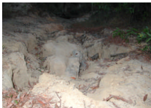
Figure 3.13: Results of poorly located and drained roads
